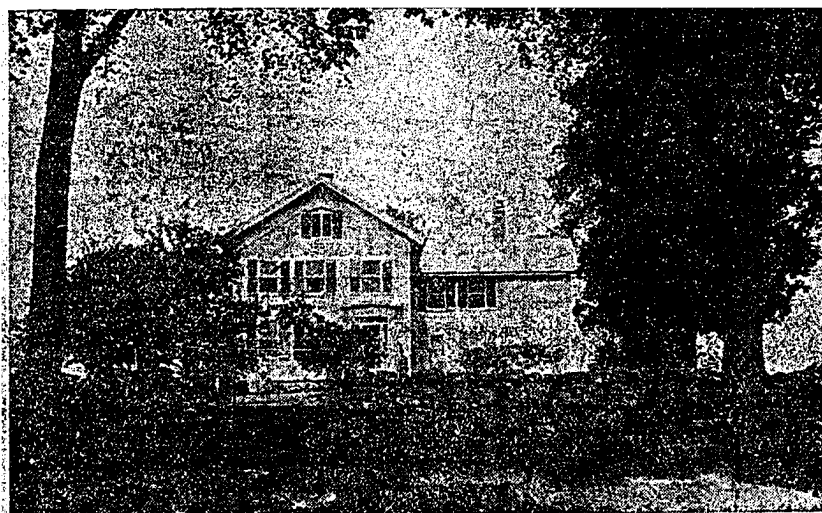
ADMINISTRATION BUILDING FROM ENTRANCE GATE ON THE ROAD
